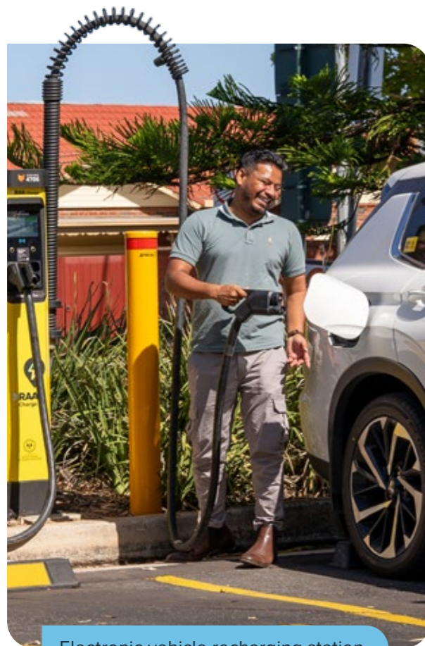
Electronic vehicle recharging station
