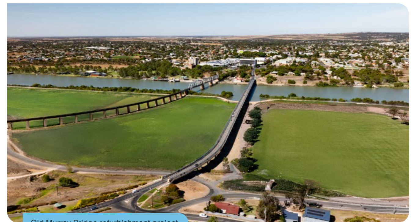
Old Murray Bridge refurbishment project
